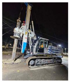
CCUR IV soil mixing crew performing soil mixing columns for groundwater control and excavation support for new underground utility construction
