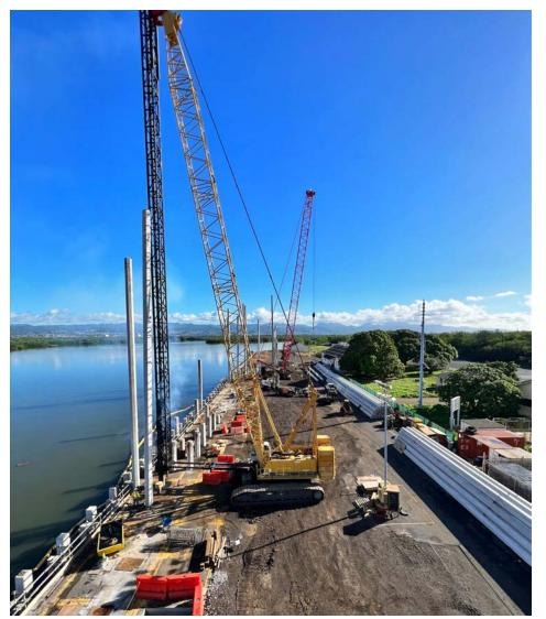
Pile driving crane preparing to drive a precast prestressed concrete pile at Ammunition Wharf W2
