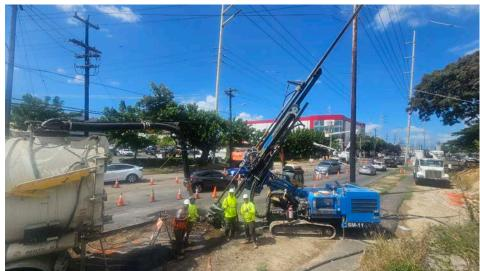
CCUR IV jet grouting crew performing "battered" jet grouting columns under existing major utilities for groundwater control and excavation support
