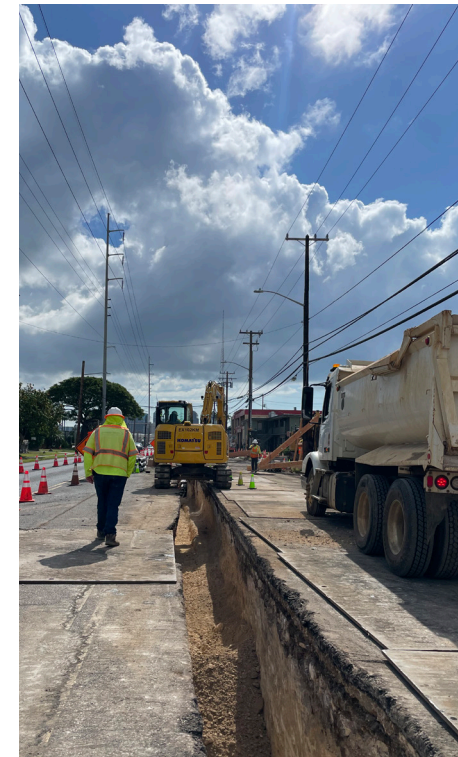
CCUR IV day-shift team performing excavator trenching
