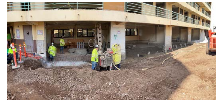
Building 502 - Structural Micropile Installation
