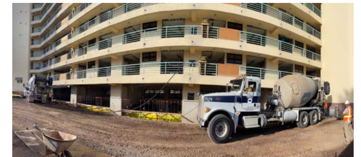
Building 502 - Shearwall Construction
