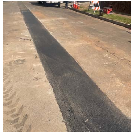
Pipe installation and temporary paving work for the Pearl City Water System Improvements Project
