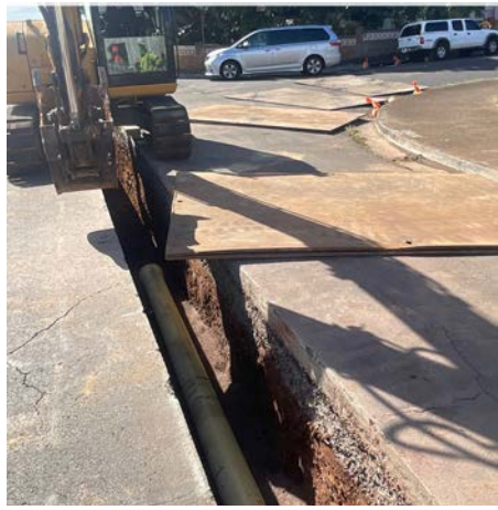
Pipe installation and temporary paving work for the Pearl City Water System Improvements Project
