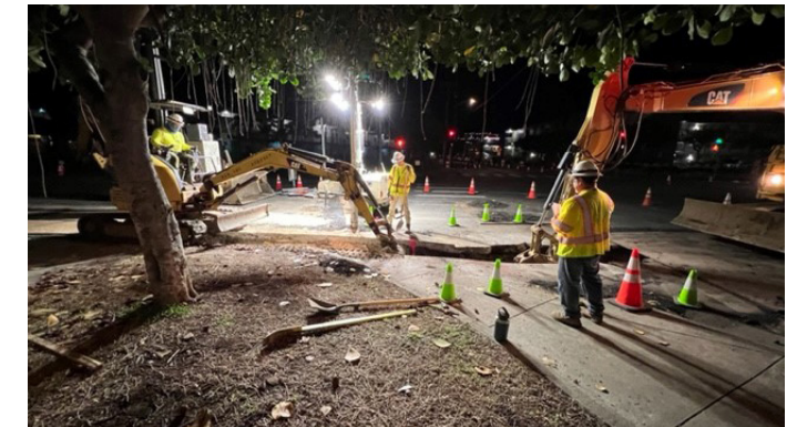
CCUR IV night-shift team trenching with a backhoe
