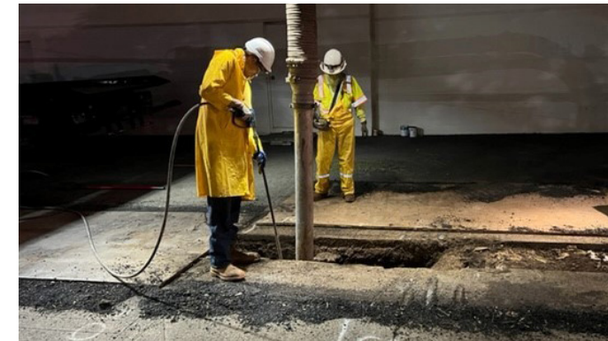
CCUR IV night-shift team potholing with a vacuum truck
