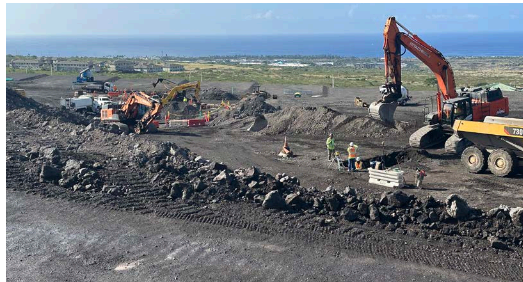
Hitachi 470 excavator installing sewer lateral at Laiopua Village 4 Phase 2 - Hema
