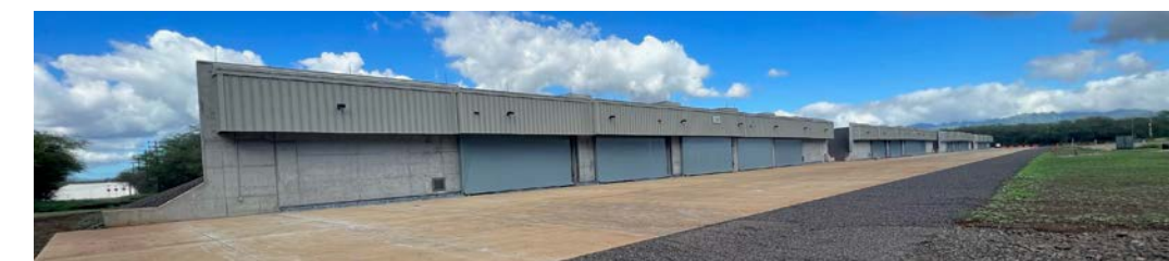
Angled view of all four newly constructed magazines
