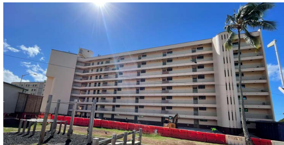
Building 502 - North Face of West Wing; Entry to Units
