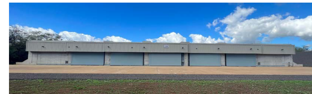
Front view of one of the new Type D Box magazines
