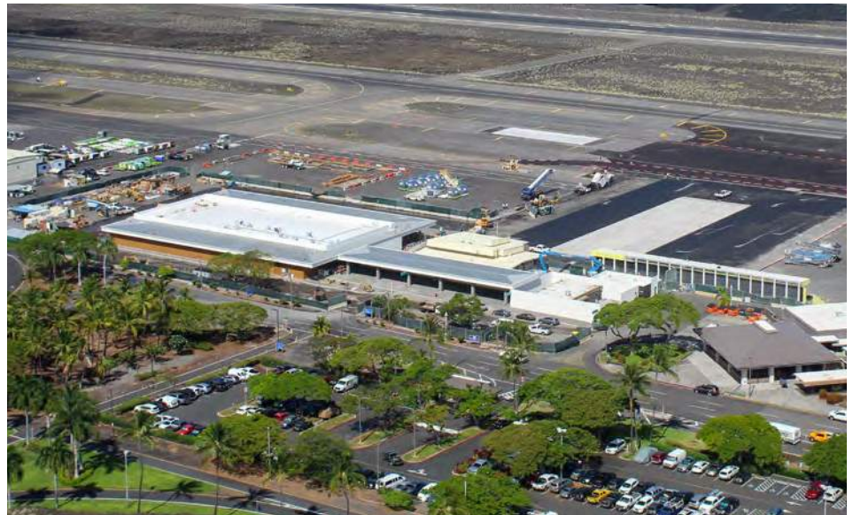
Aerial view of KOA Federal Inspection Services (FIS) Building
