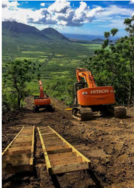
Replacement of mountain line at NAVMAG Lualualei
