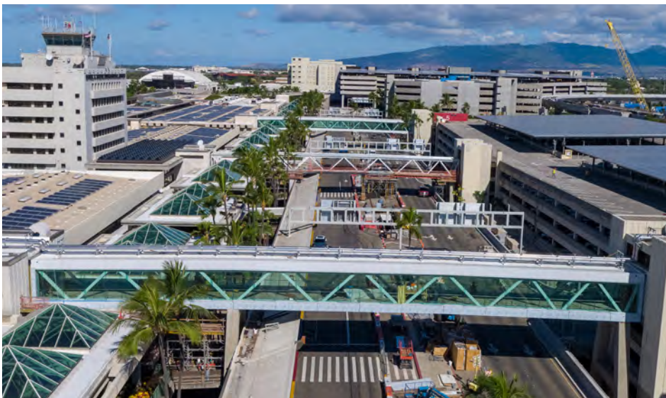
View of Pedestrian Bridge progress at Daniel K. Inouye International Airport
