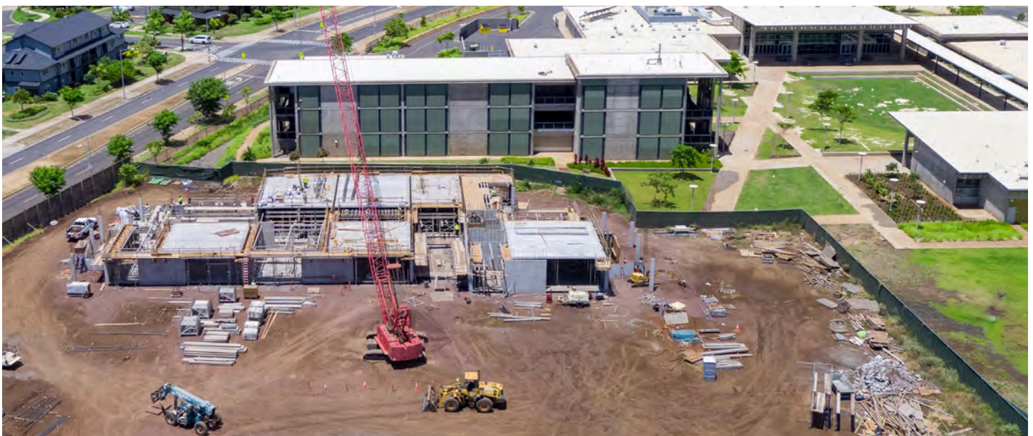
Phase 2 of Honouliuli Middle School under construction
