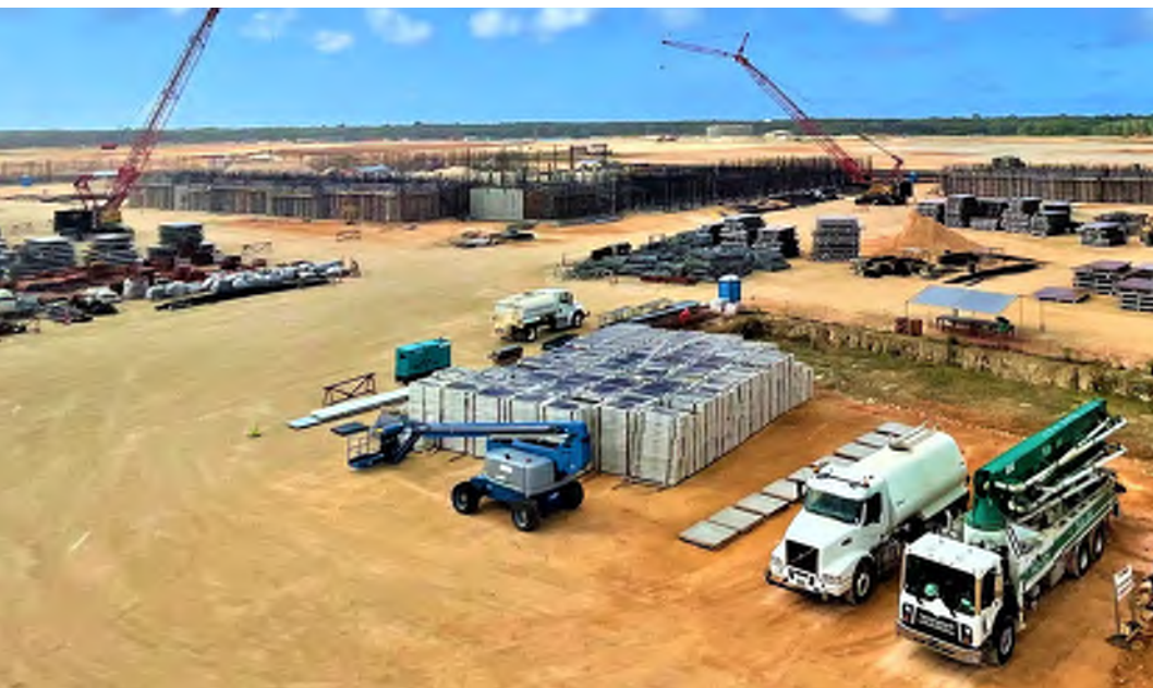
Nan, Inc. constructing BEQ D and F
