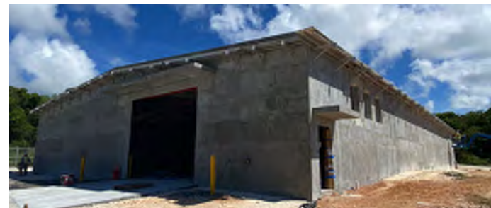
P295 Ordnance Operations Facility
