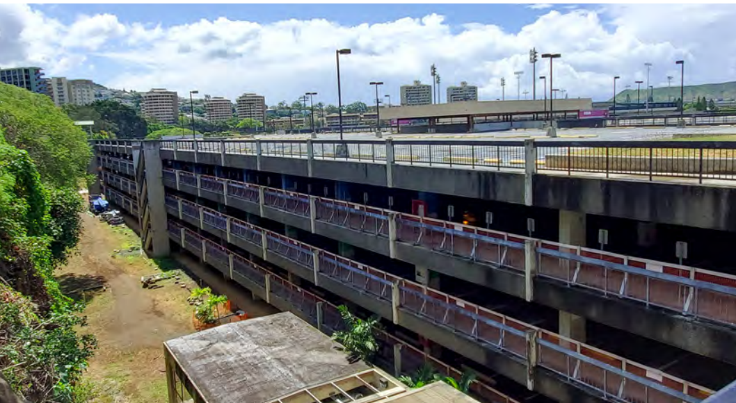
Guardrail Repairs at University of Hawaii Manoa's Parking Structure
