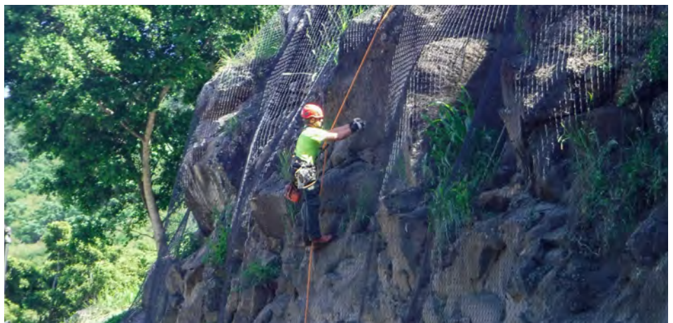
Rockfall protection at Red Hill Tunnel
