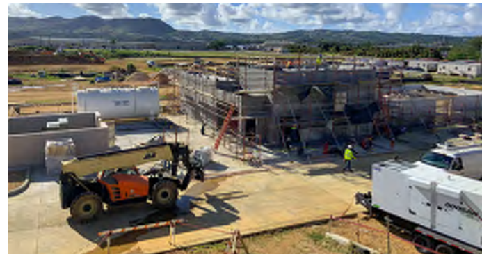
Construction of APRA Medical Dental facility
