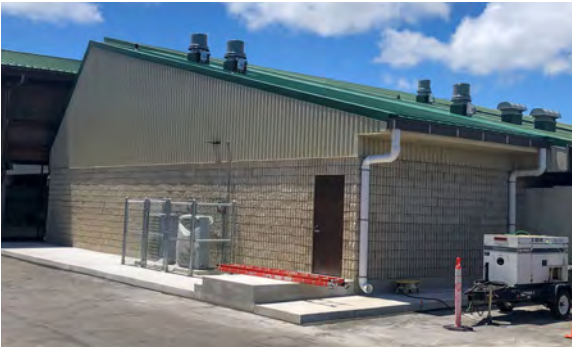
Exterior of Hilo International Airport restroom
