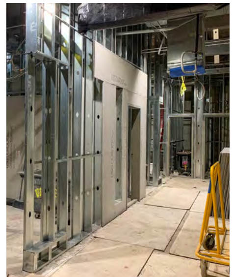
Construction of HNL Restroom Improvements
