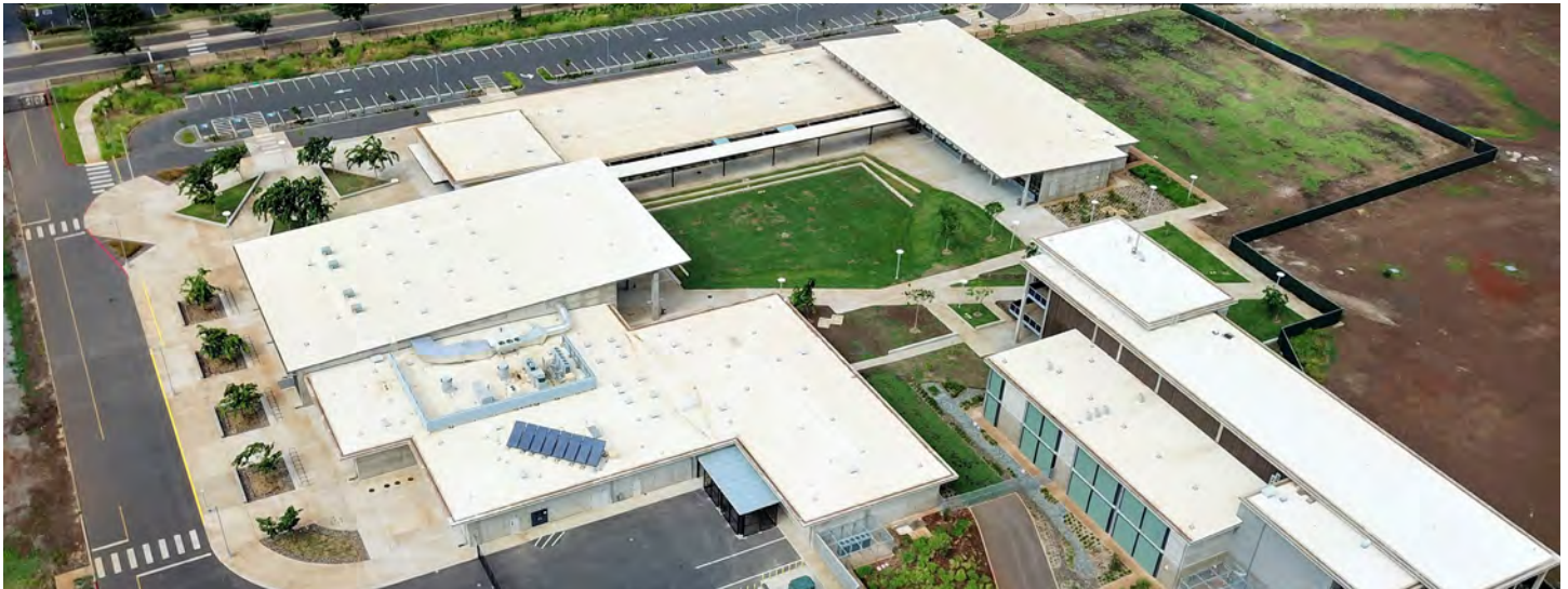
Completed phase 1 of Honouliuli Middle School
