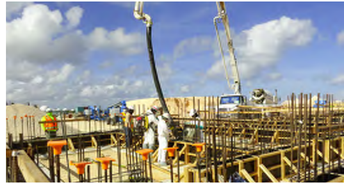
The CNJV crew pumping concrete at BEQ H
