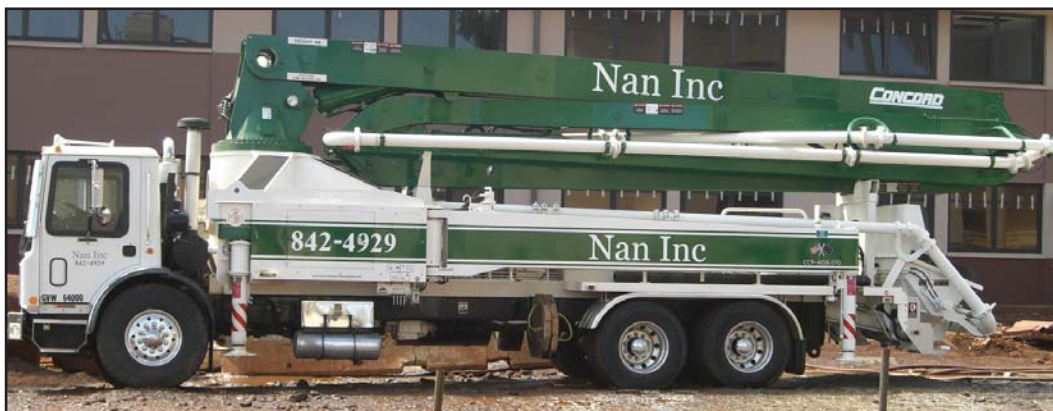
Nan, Inc.'s newest Mack concrete pump truck goes to work.
