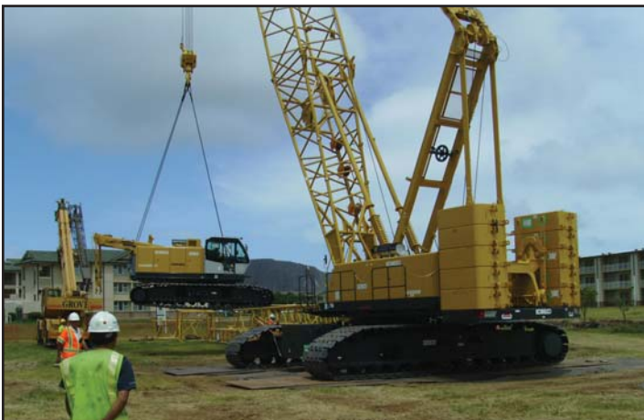
The new Kobelco CK2000 moving and assembling the CK1000.
