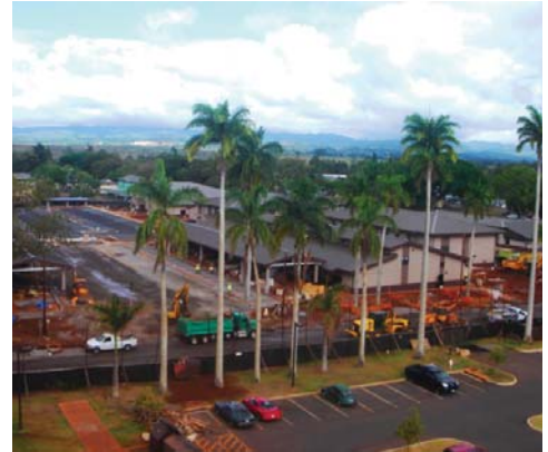
COF13 Hardstand Readiness Building & Administration Building
