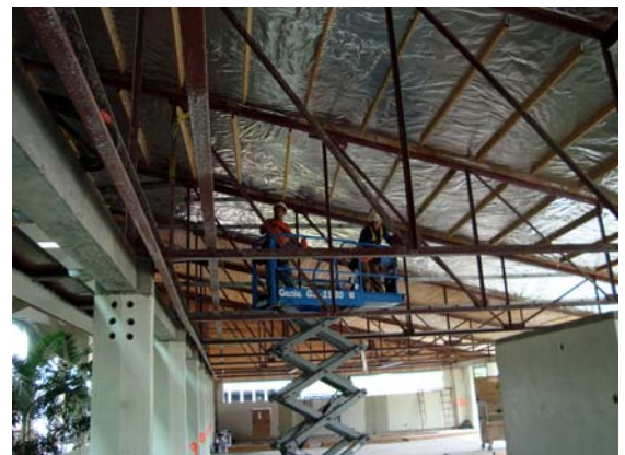
Ongoing work within the Hawaii County Building Renovation project
