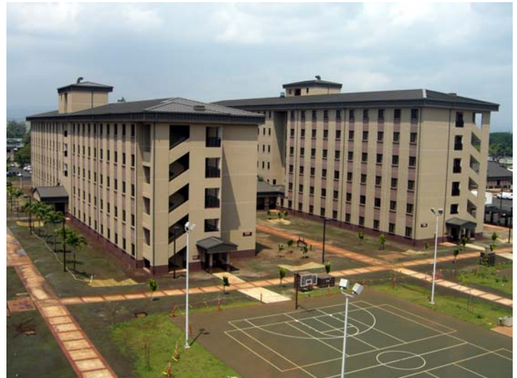
Completed Five-Story (left) and Six-Story (right) Barracks
