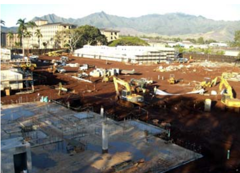
Current 2F2/2G project site
