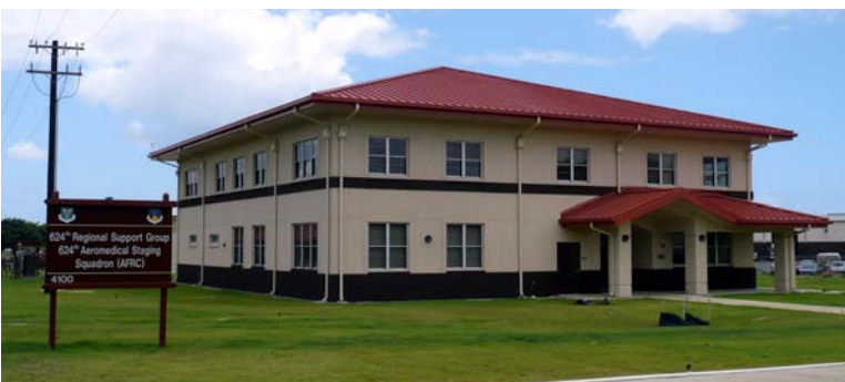
Completed Hickam Consolidated Training Facility
