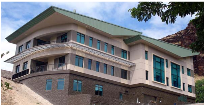
Completed Weinberg Family Medical Center
