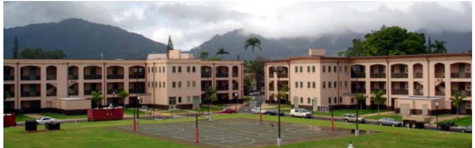
Buildings 550/551 and the Courtyard of Quad E
