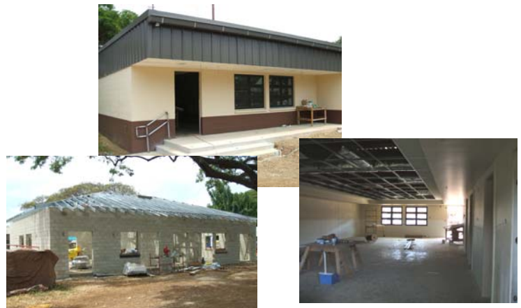
Pictured (clockwise, from top): Exterior and Interior of Child Care Development Center, Bldg. 1654; and Child Care Development Center, Bldg. 1597.
