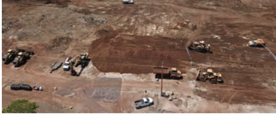
Photos, from the top: Mass excavation underway at 24 acre site; Preparing for ground blessing ceremony, February 7, 2019; Nan, Inc. Vice President Frank Okimoto (fourth from left) next to Honolulu Mayor Kirk Caldwell at ground blessing ceremony; Existing Honouliuli wastewater treatment facility
